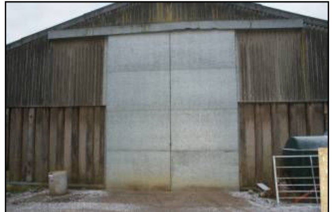
Fig 3: Example of good fitting doors that will prevent access to badgers.
