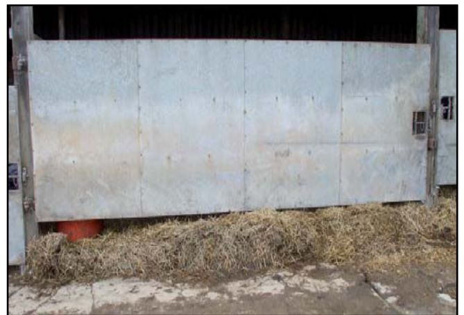
Fig 4: Example of a gate allowing access to badgers.
