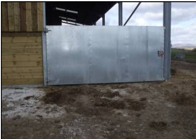
Fig 7: In accordance with FERA advice, gaps under gates should be less than 10cm to help prevent wildlife gaining access.
