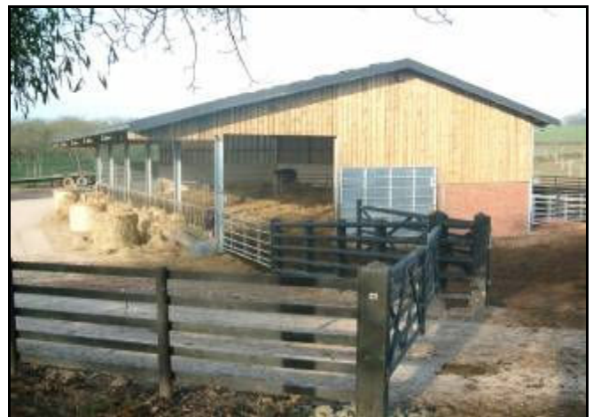
Fig 4: An example of an isolation unit.
